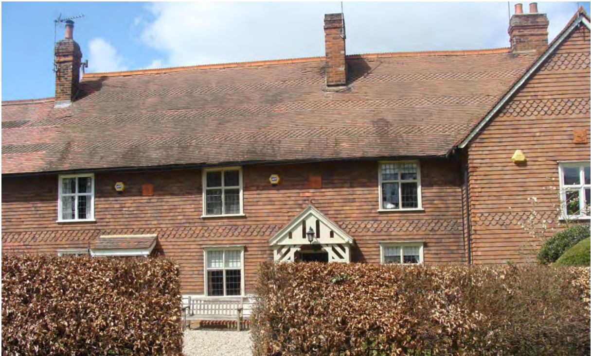
Picture 1.12 Nos. 1,2 and 3 Church End, 17th century in origin with distinctive 19th century scalloped tile detailing to walls and roof
