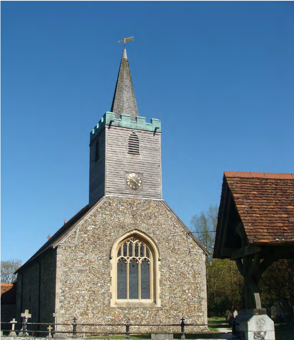
Picture 1.11 Great Canfield church with its weather boarded 15th century bell tower and 19th century spire
