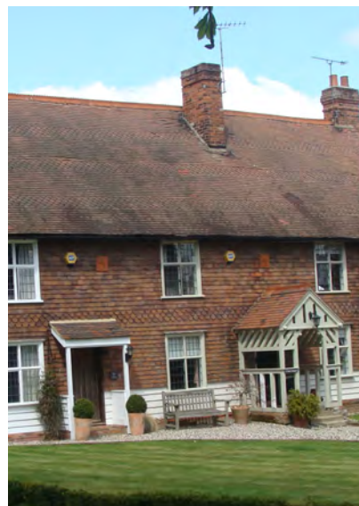
Picture 1.5 Alternating bands of plain and scalloped tiles to the walls and roof of Nos. 1 to 3 Church End lend great decorative effect to these timber-framed dwellings
