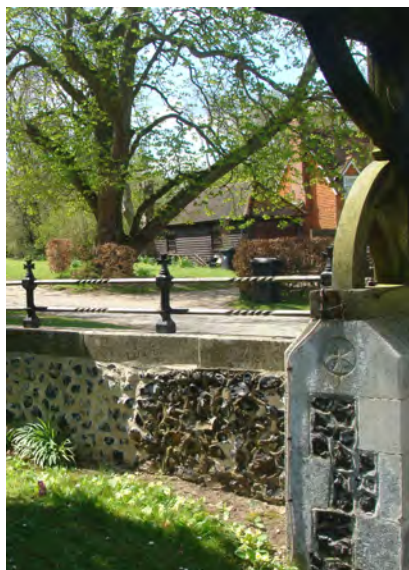
Picture 1.4 Decorative iron railings set on half walls surrounding St Mary's Church
